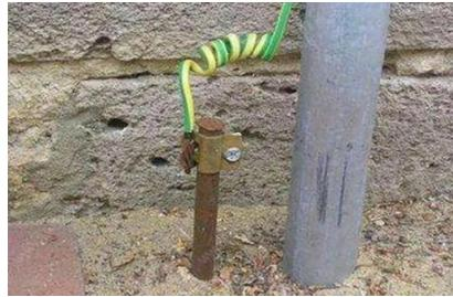
Connect the other end of the grounding wire to a reliable grounding post.
